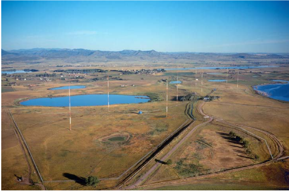
An aerial photograph of the site shared by WWV and WWVB near Fort Collins, Colorado, taken during the 1990s. The relatively small WWV antennas are not visible from the angle of this photograph, but the eight large towers support the massive WWVB antenna array visible in the foreground.
