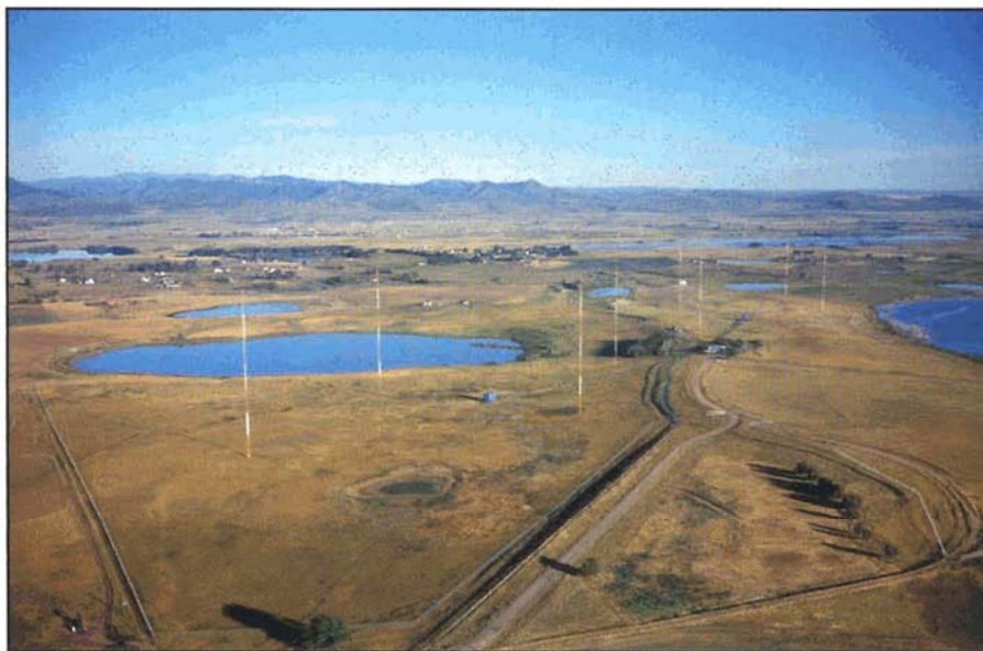
An aerial photograph of the site shared by WWV and WWVB near Fort Collins, Colorado, taken during the 1990s. The relatively small WWV antennas aren't visible from this angle, but the eight large towers support the massive WWVB antenna array.
