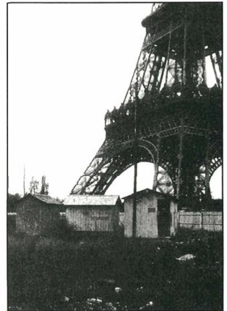
A photograph of the Eiffel Tower, published in 1909 prior to the start of the time broadcasts, which began in May 1910. It shows the small buildings at the base of the tower that housed the radio station equipment.
