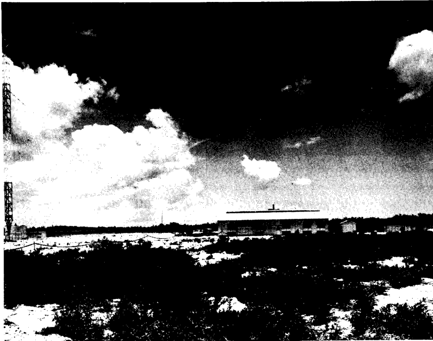
Figure 6.2 Jupiter Station after completion.
