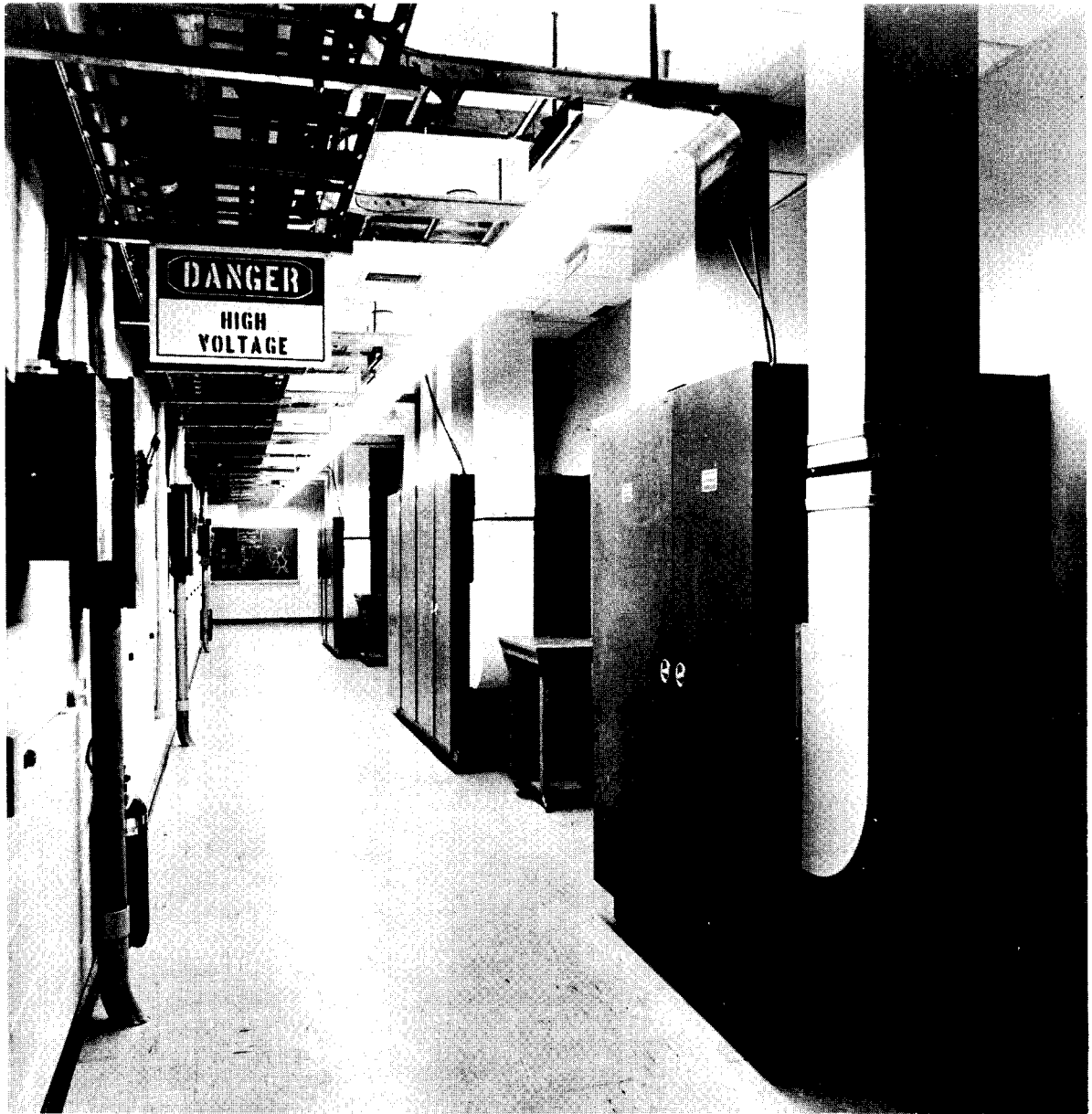
Figure 7. The south corridor of the building behind the transmitters, showing overhead cable trays, power line disconnect switch, and air ducts to the transmitters.
