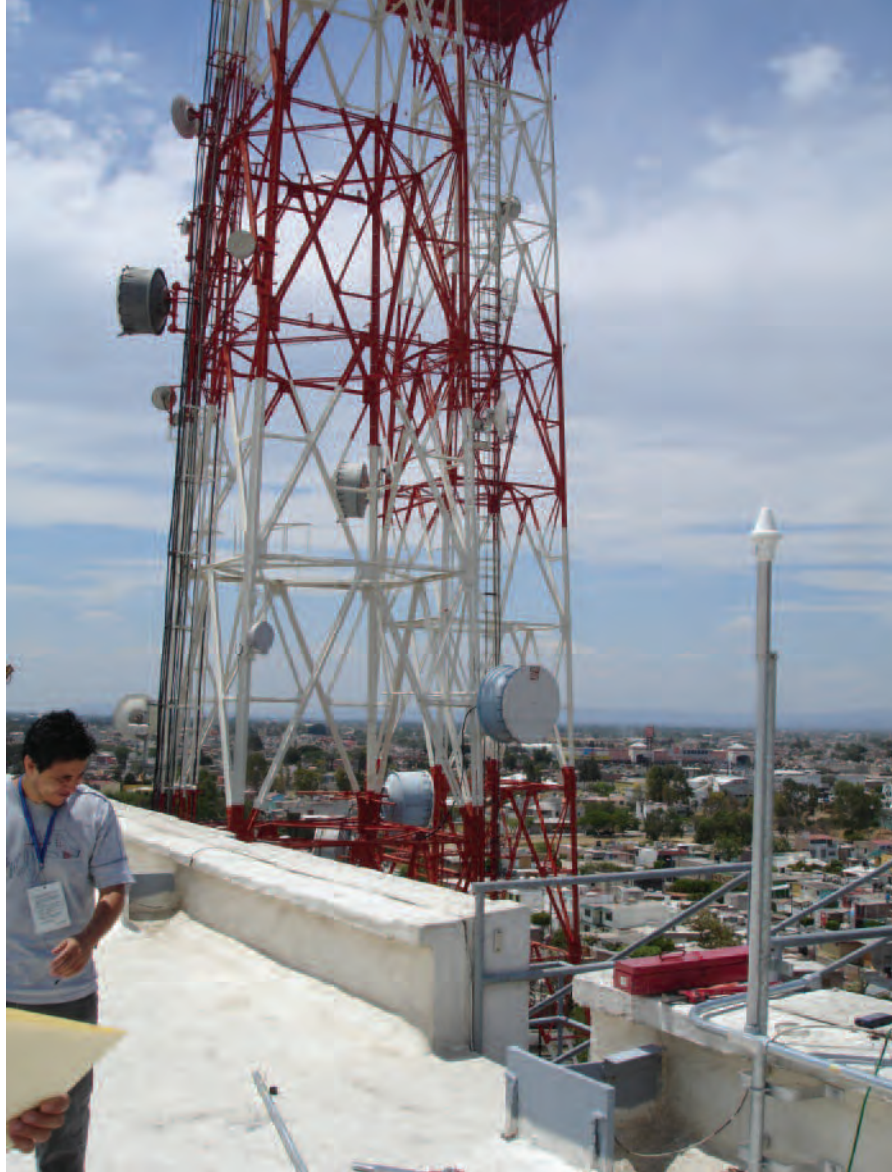
Figure 8. GPS installation at a TELMEX site.
