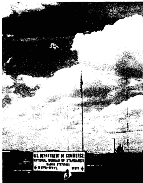
WWVB/WWVL transmitter building and antennas.
